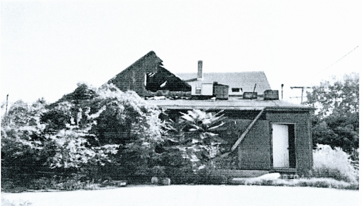
PHOTO 2 (View of rear of building)
