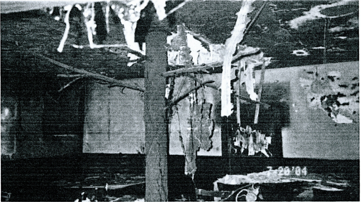
PHOTO 5 (First Level Front Dining Room - Typical Condition)
