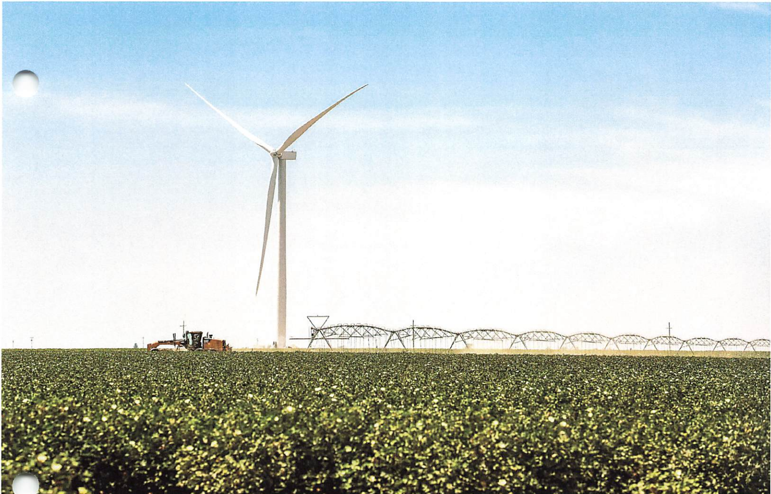
The 80-MW Lorenzo Wind Energy Center in Texas.
