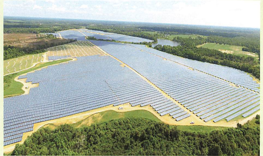
The 51-MW Live Oak Solar Energy Center in Georgia.
