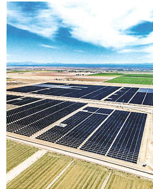
The 20-MW Pinal Central Solar Energy Center in Arizona was NextEra Energy Resources' first project to pair solar energy with an on-site, state-of-the-art 10-MW battery storage system.
