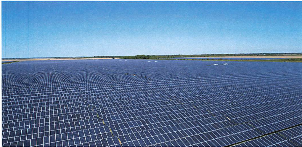
The 81-MW Stuttgart Solar Energy Center in Arkansas.
