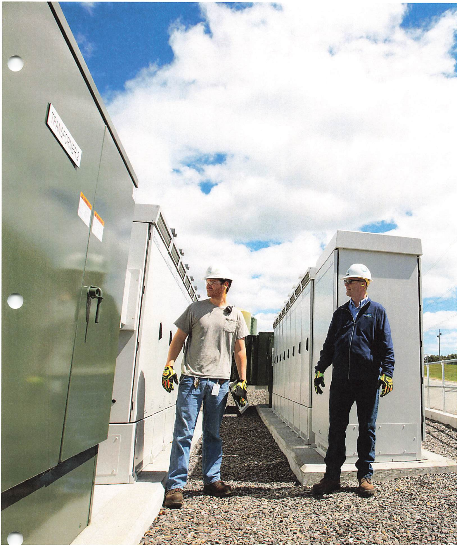
Employees at the 16-MW Casco Bay Energy Storage Center in Maine.
